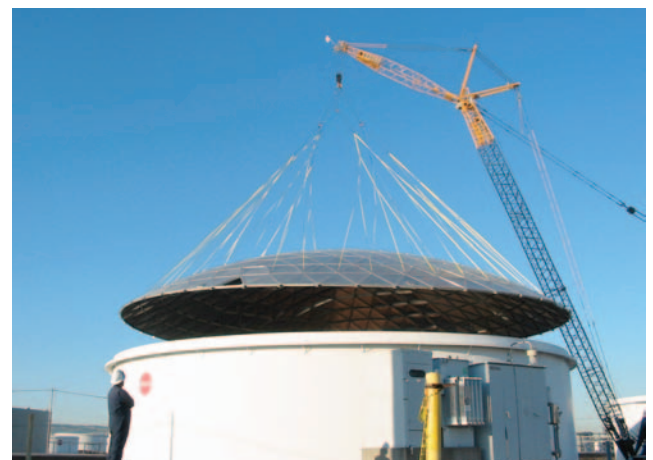
Geodesic dome roof is installed on a tank
